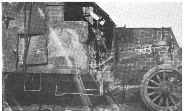
Armored Pierce truck, disguised as brick wall, hit by shell
